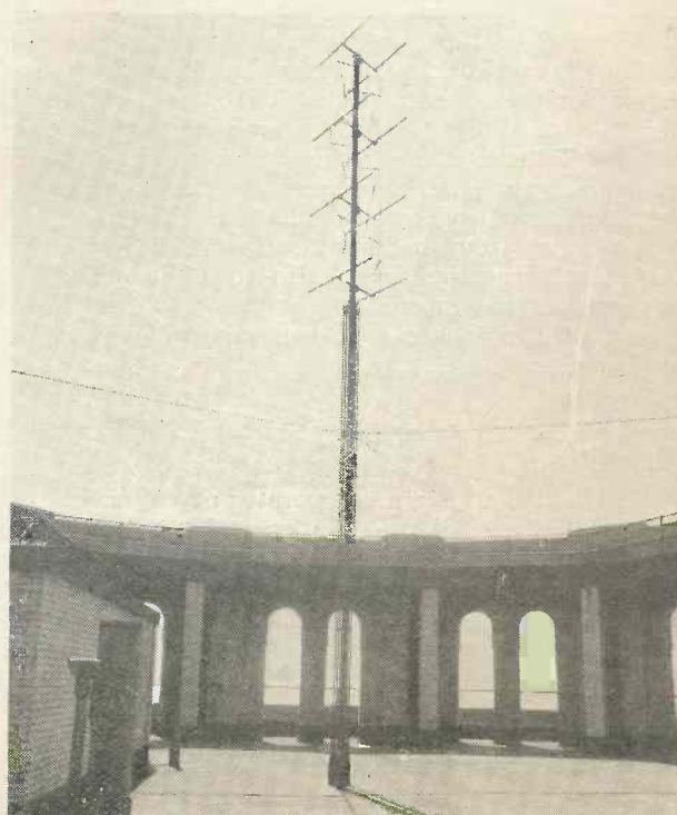
The ultra-short wave aerial on top of an office building in New York.
